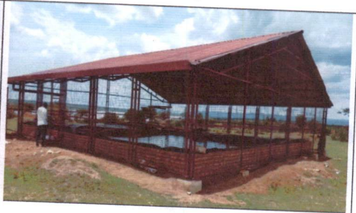
Solar irrigation system at Byimana site
