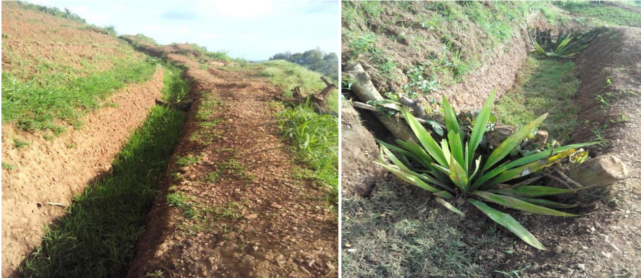
Figure 8: Infiltration trenches to reduce runoff
