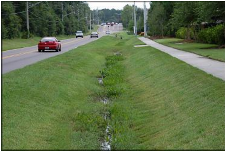
Figure 9: Swales like the above is good for runoff infiltration (Source: https://brocku.ca/unesco-chair/2020/01/27/meopar-blog-swales-the-silent-stormwater-sweepers/ )
