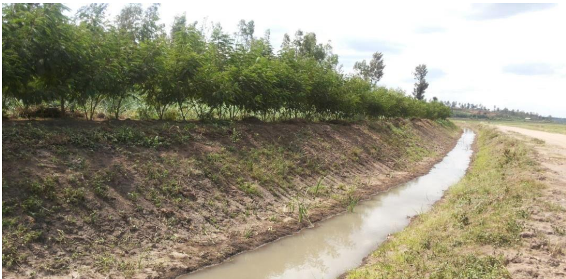
Figure 6: Grasses planted on the ridges helps to stabilize it and prevent erosion
