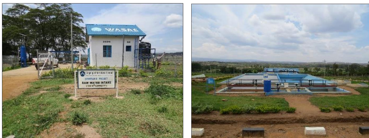
Figure 38. Raw water intake station (left) and water treatment plant (right), established by WASAC, along the banks of the Muvumba River in Nyagatare District. Source: Kevin Emslie, 14 February 2018.
