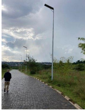
Recessive paving, no patterns, strong herringbone bonds for coping with curvilinear routes
