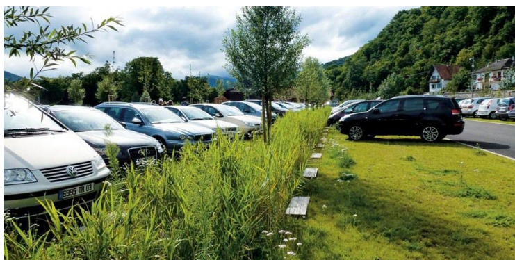
Reinforced grass parking areas with central drainage swales are more ecologically friendly
