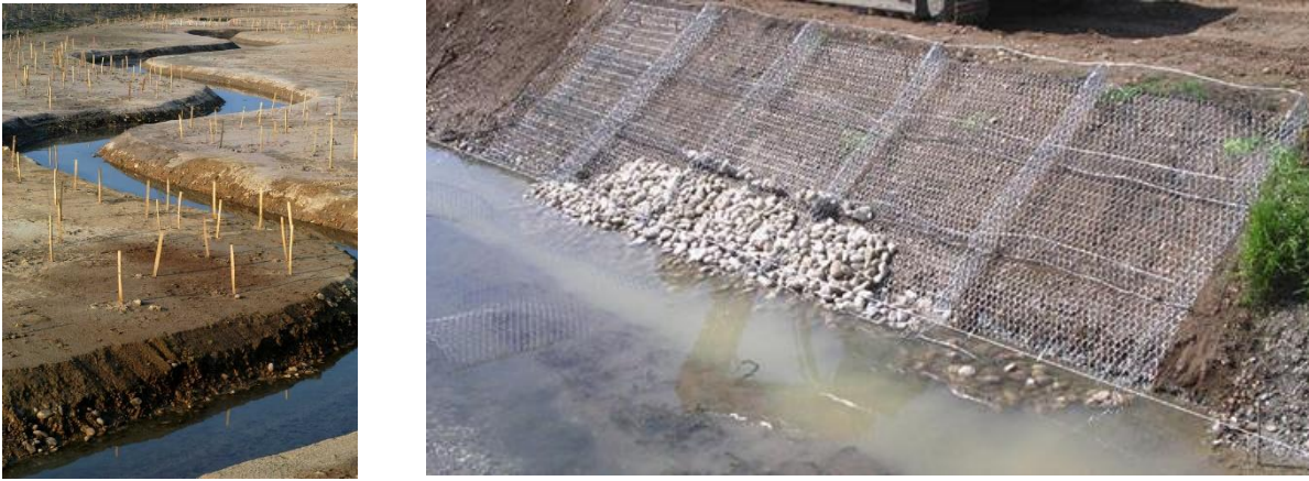
FIGURE 5-68: EXAMPLE OF RIVER MEANDERING AND EXTERNAL BANKS PROTECTION WITH GABIONS
