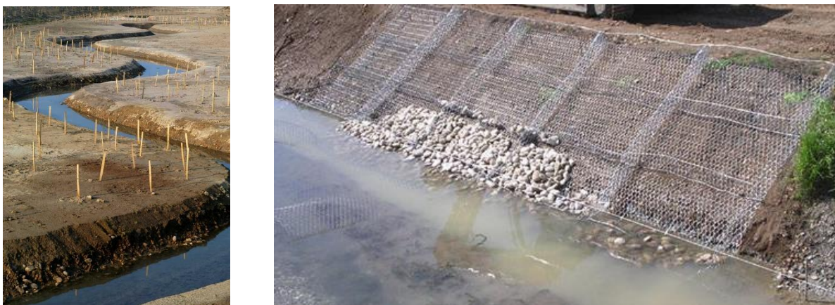
FIGURE 5-90: EXAMPLE OF RIVER MEANDERING AND EXTERNAL BANKS PROTECTION WITH GABIONS
