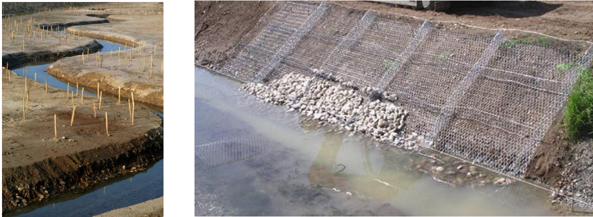
FIGURE 5-52: EXAMPLE OF RIVER MEANDERING AND EXTERNAL BANKS PROTECTION WITH GABIONS
