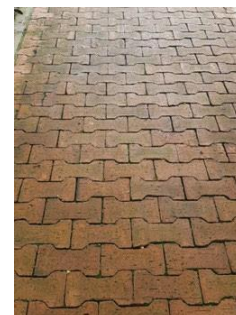
Baked red brick paving blocks, interlocked, but this pattern may be difficult around bends
