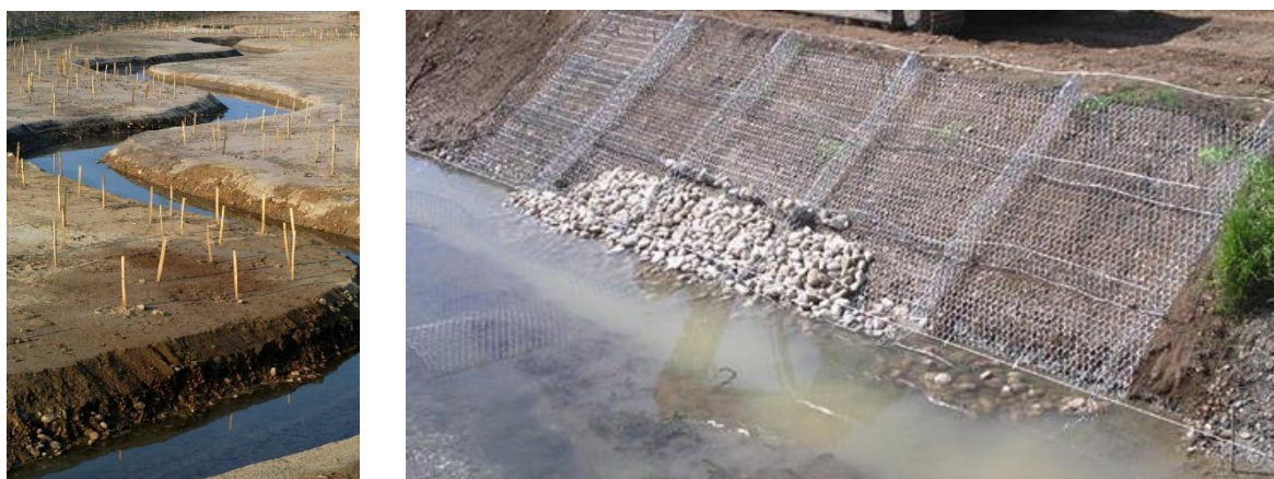
FIGURE 5-30: EXAMPLE OF RIVER MEANDERING AND EXTERNAL BANKS PROTECTION WITH GABIONS
