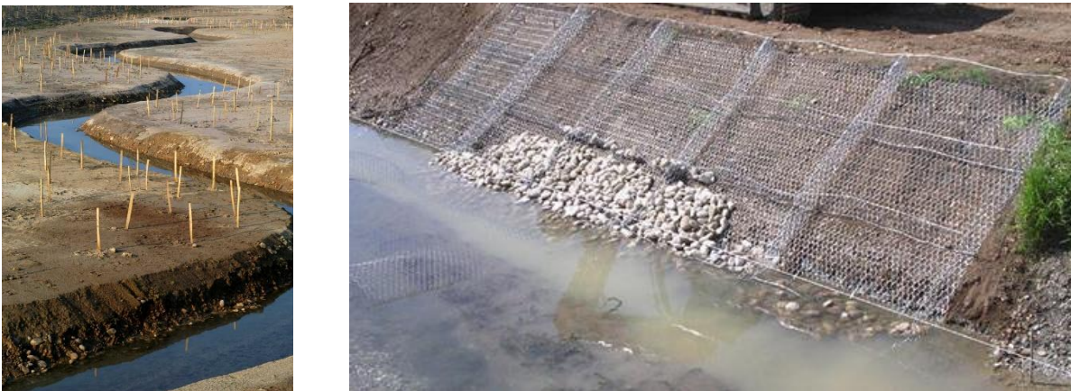
FIGURE 5-105: EXAMPLE OF RIVER MEANDERING AND EXTERNAL BANKS PROTECTION WITH GABIONS
