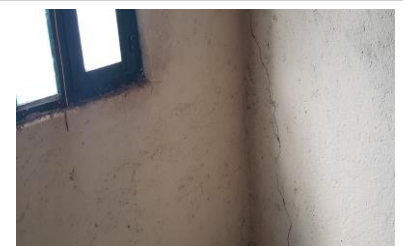
Cracks in house in Nyenyeri claimed to be a vibration effect.
