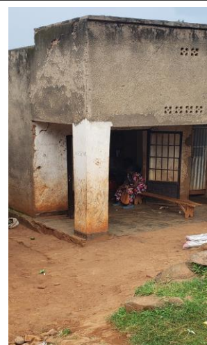
Cracks on house in Nyenyeri claimed to be a vibration effect.
