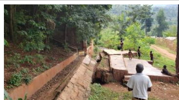
Stormwater Discharge channel & collapsed wall
